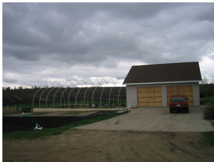
Greenhouse prior to final completion.
